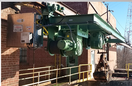
Left: Two independent hoists in a common frame. Right: Gearboxes mounted at different elevations to allow for better cable management.
